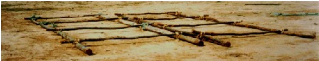
Assemble tower sections on the ground, and then use guy ropes to lift the sections, and to hold them in position, until they can be connected with cross-poles.
