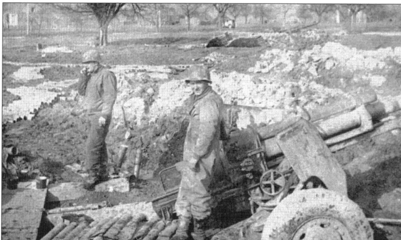
The towed tank destroyer battalions were frequently used for other roles in the 1945 fighting, sometimes as indirect artillery. Here, the 824th Tank Destroyer Battalion has their 3in guns emplaced for artillery fire missions during February 1945. The fiberboard packing tubes from the ammunition have been used to fashion a "corduroy" road and work area in the mud near the gun. (L. Kreiser collection, MHI)
